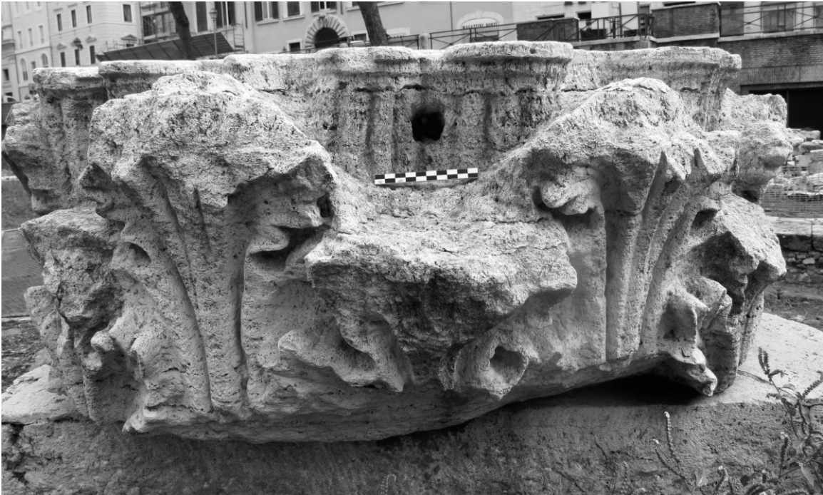
Fig. 5: The lower half of a capital from Temple B in Largo Argentina vowed in 101 BCE. Note that the highest acanthus leaves rise just to the plane of the seam between lower and upper capital halves (photo by author).
