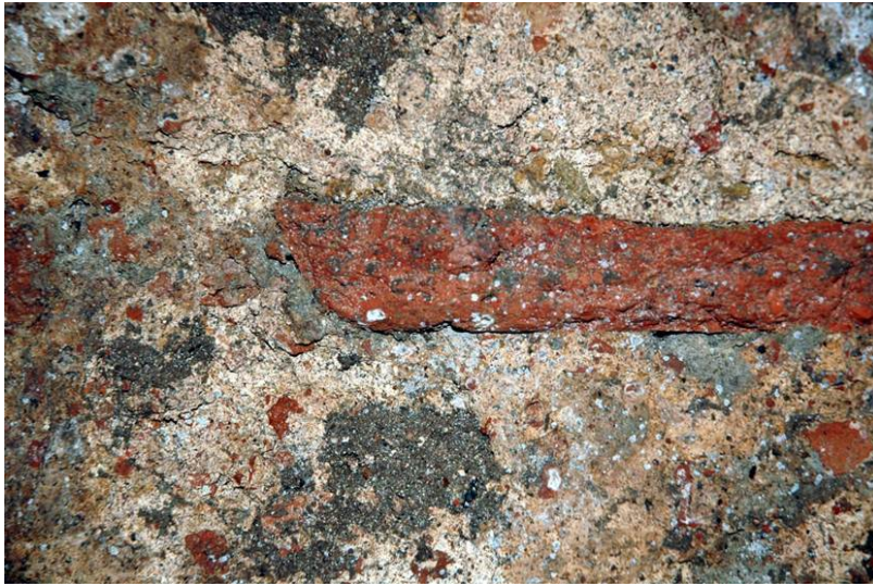
Fig. 11: Constantinople, ruins of an unknown Byzantine building under the carpet shop “Sedir” next to the Hippodrome. Brick with a beveled edge.
