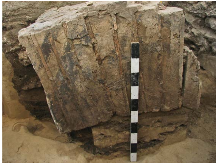
Fig. 4: Tithe Church. Masonry unit of thin brick on lime mortar.
