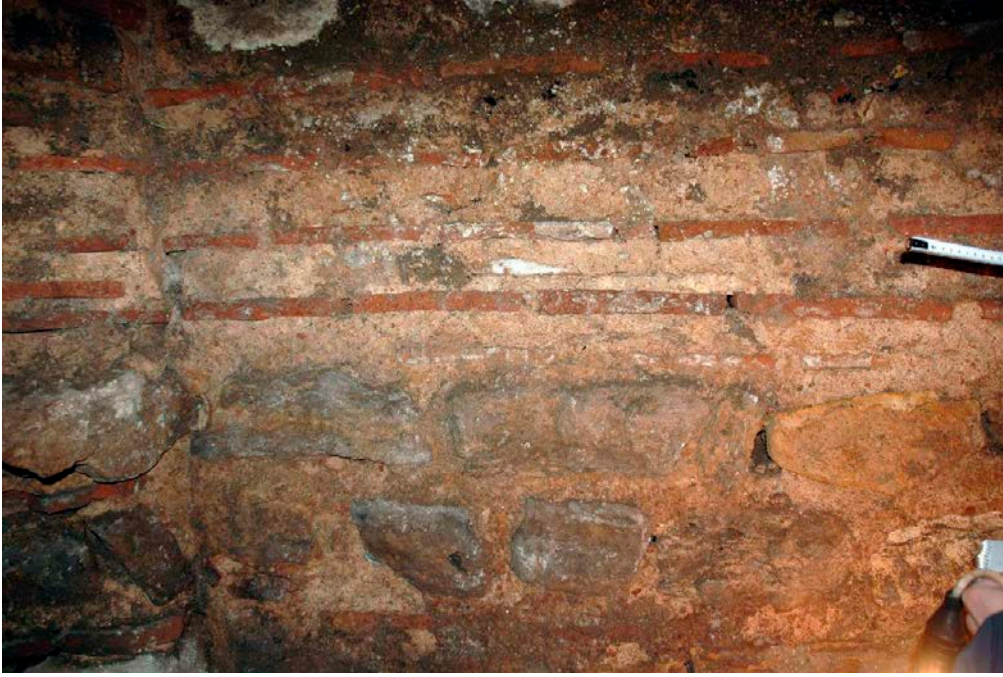
Fig. 10: Constantinople, ruins of an unknown Byzantine building under the carpet shop “Sedir,” next to the Hippodrome. Masonry with the concealed course technique.
