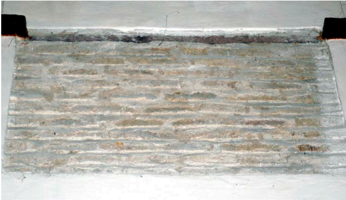
Fig. 24: Chernigov, Cathedral of Saints Boris and Gleb. Masonry using the equicourse technique.
