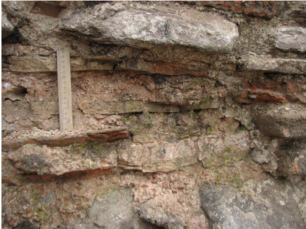
Fig. 7: Tithe Church. Foundation masonry with thin brick and stone.
