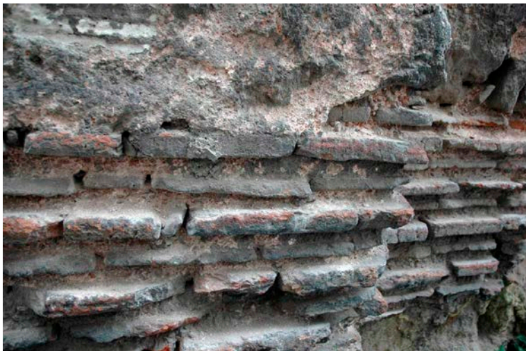
Fig. 8: Constantinople, Church of Pantokrator. Bricks with beveled edges in the concealed course technique masonry.
