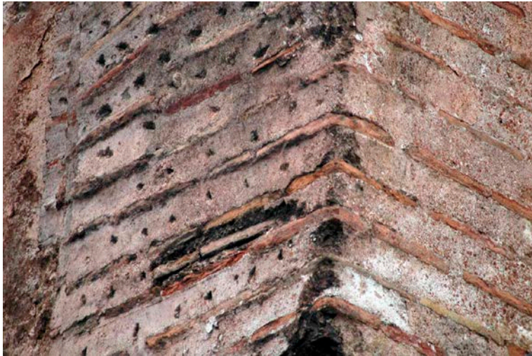
Fig. 9: Constantinople, Church of the Pantokrator. Masonry with the concealed course technique.
