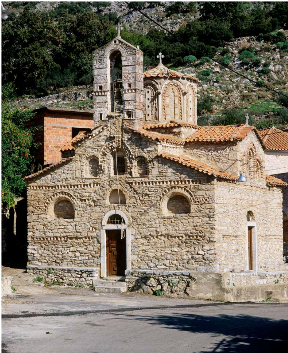
Fig. 2. Church of the Soterias, view from west after its masonry was revealed (author).
