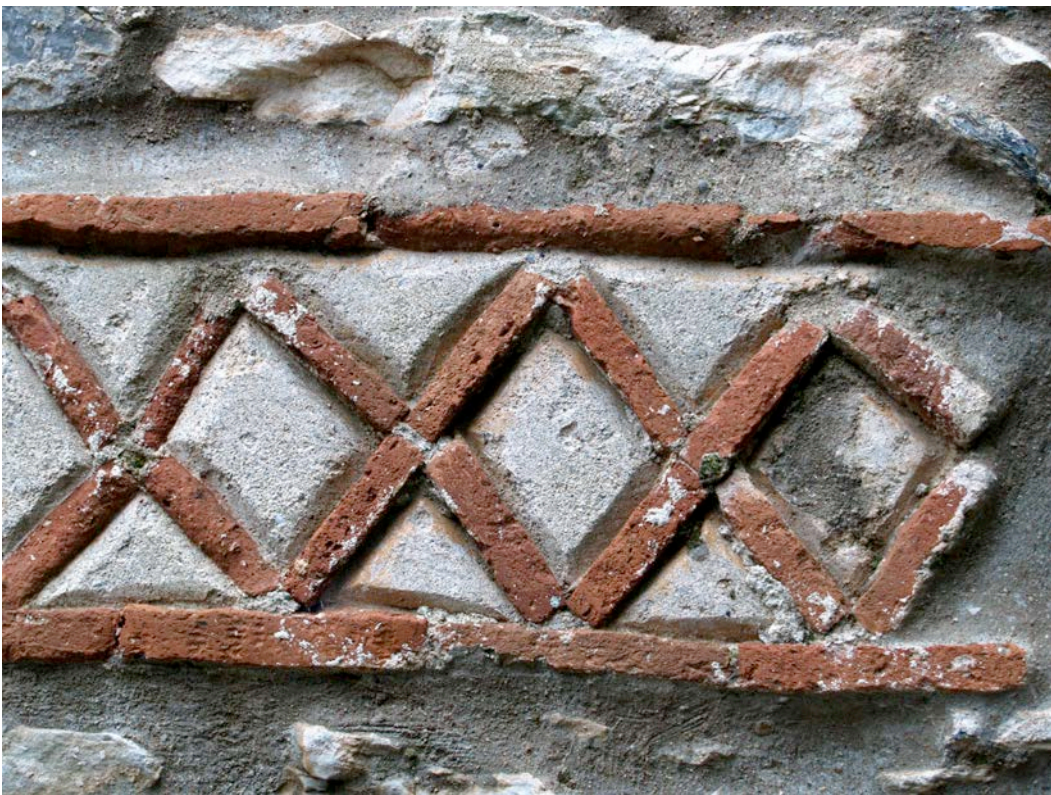
Fig. 9. Detail of the application of mortar in the brick decoration of the Soterias church (author).
