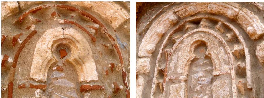
Fig. 11. Detail of the blind arches adorning the diagonal sides of the dome's drum (author).
