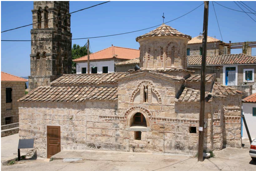
Fig. 27. Church of St. Nicholas, Prasteio, view from south (author).
