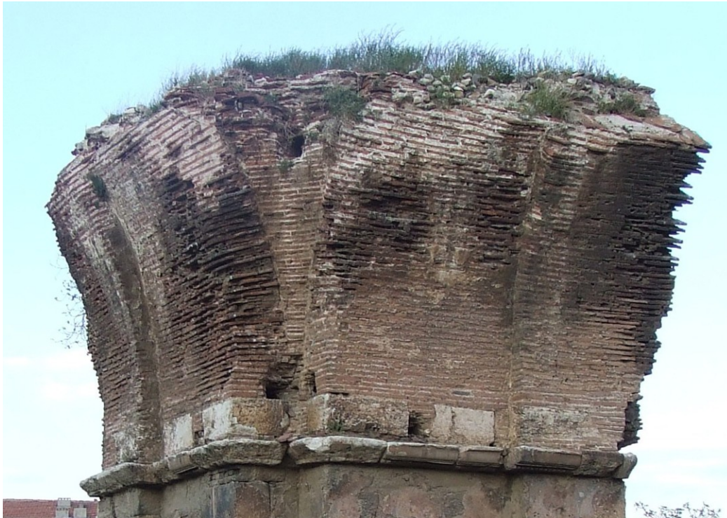
Fig. 10: Philadelphia, St. John, Detail of Vault Fragment on top of the Northeast Pier, displaying remains of a pendentive (photo by Nikolaos Karydis, 2007).
