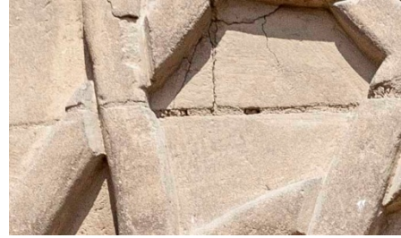
Figure 15: Mausoleum of Janibak, detail of dome showing wooden pegs (photo: B. O’Kane).
