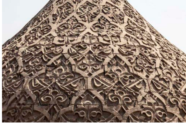
Figure 9: Qanibay complex, detail of dome (photo: B. O’Kane).
