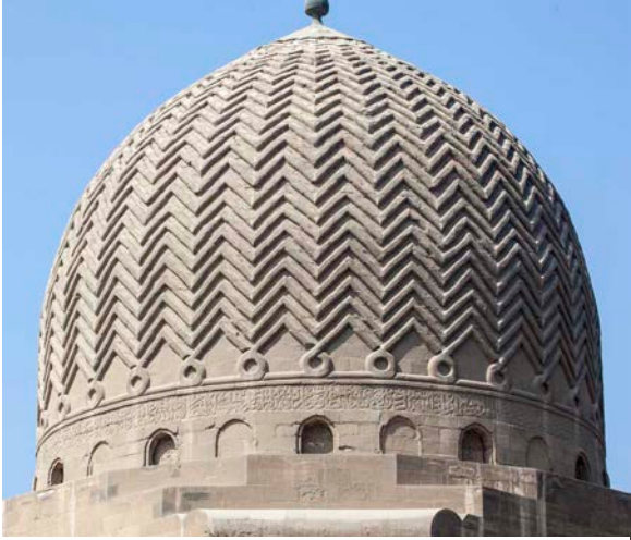
Figure 5: Faraj ibn Baquq complex, Cairo (photo: B. O'Kane).
