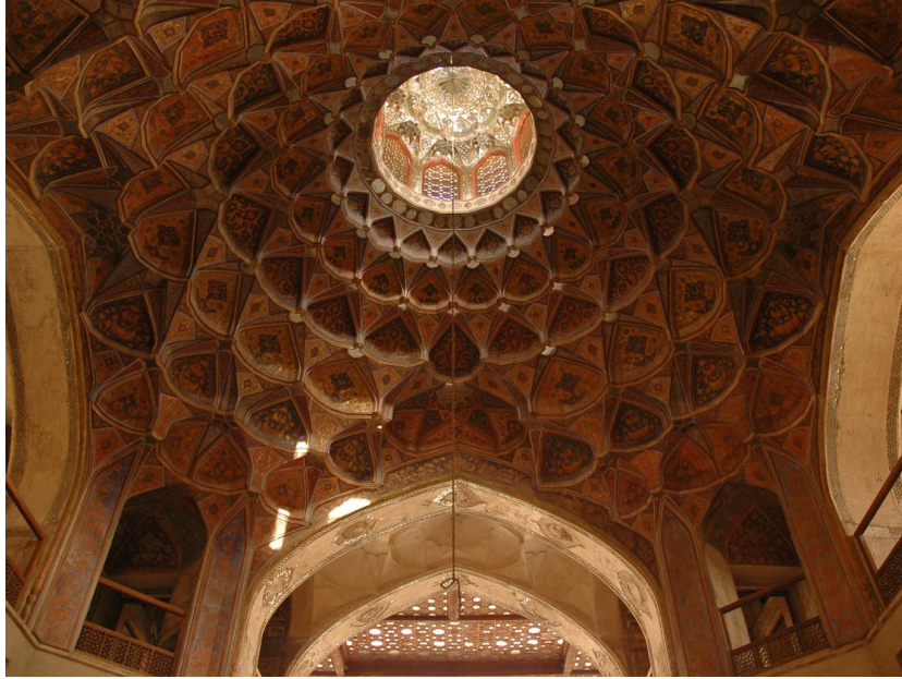
Fig. 5: Fig. 5: Hasht Behesht Palace in Isfahān. View of the alveolate ceiling of the central covered space from the inside.
