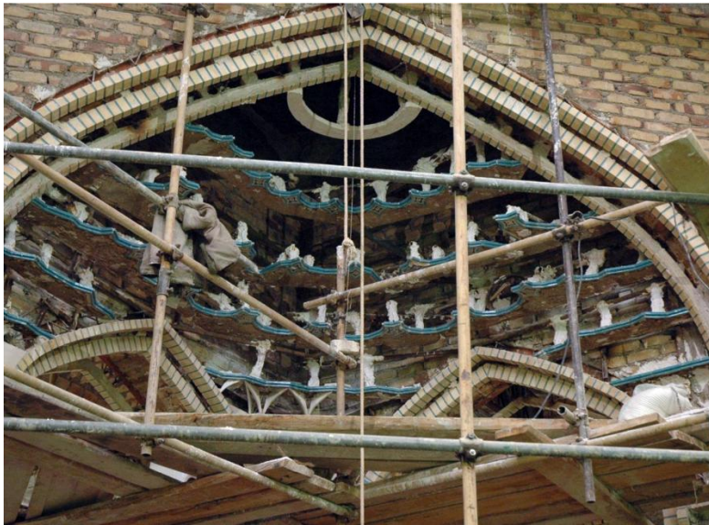
Fig. 4: Detail of the ribs sustaining the timber lintels and the ropes for the muqarnas ceiling in the Mausoleum Habib Ibn Musa in Kāshān.
