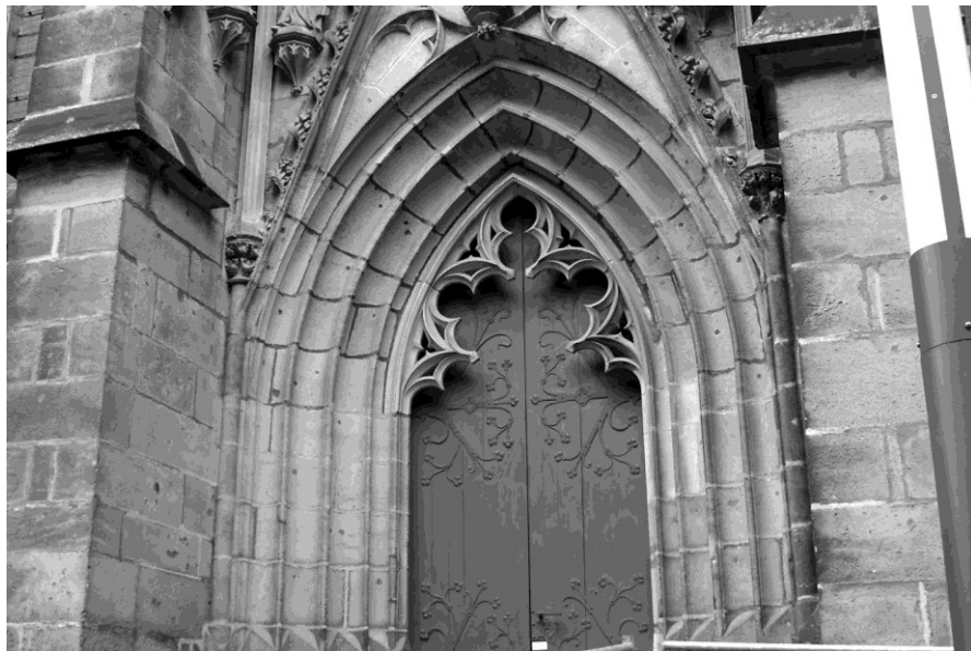
Fig. 8: Filled Lifter Holes on the Outer Walls
