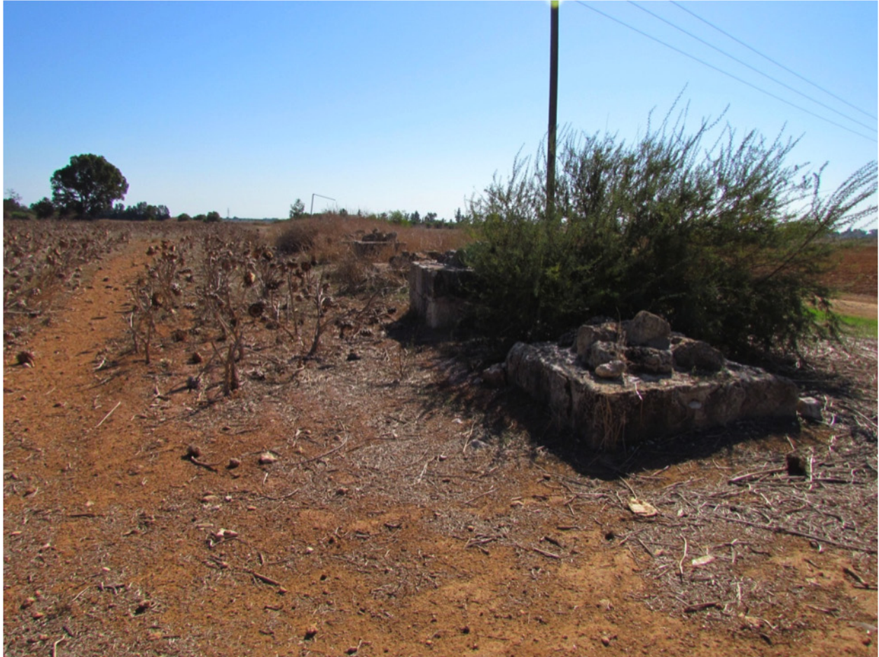
Fig. 11: Chytroi-Salamis-Constantia Aqueduct. Remains of seven piers. View eastward.
