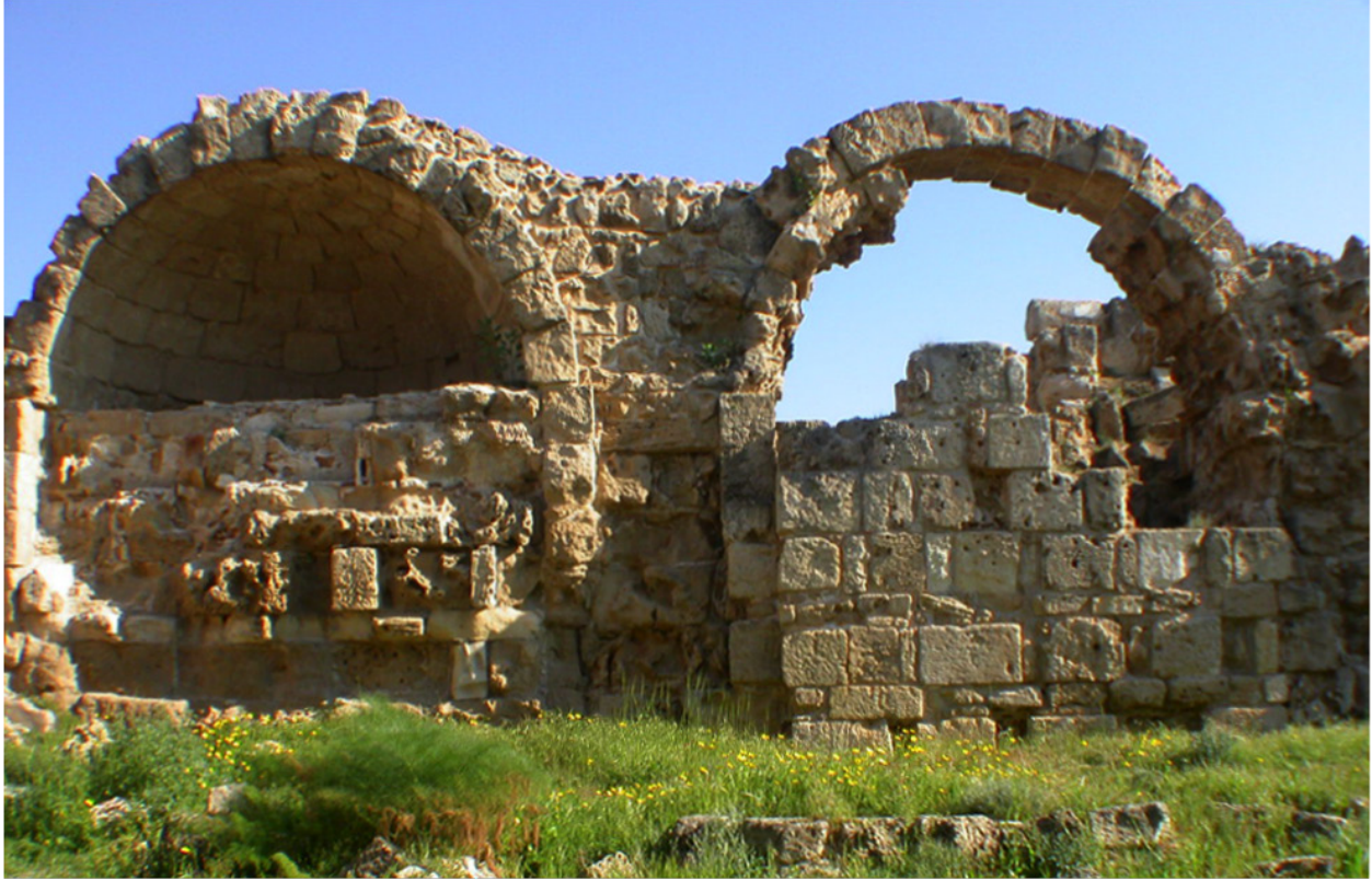
Fig. 6: Grand Baths at Salamis-Constantia. North wall of the sudatorium showing two apsidal chambers blocked-up which coincided with the construction of the flying buttresses on the other side.
