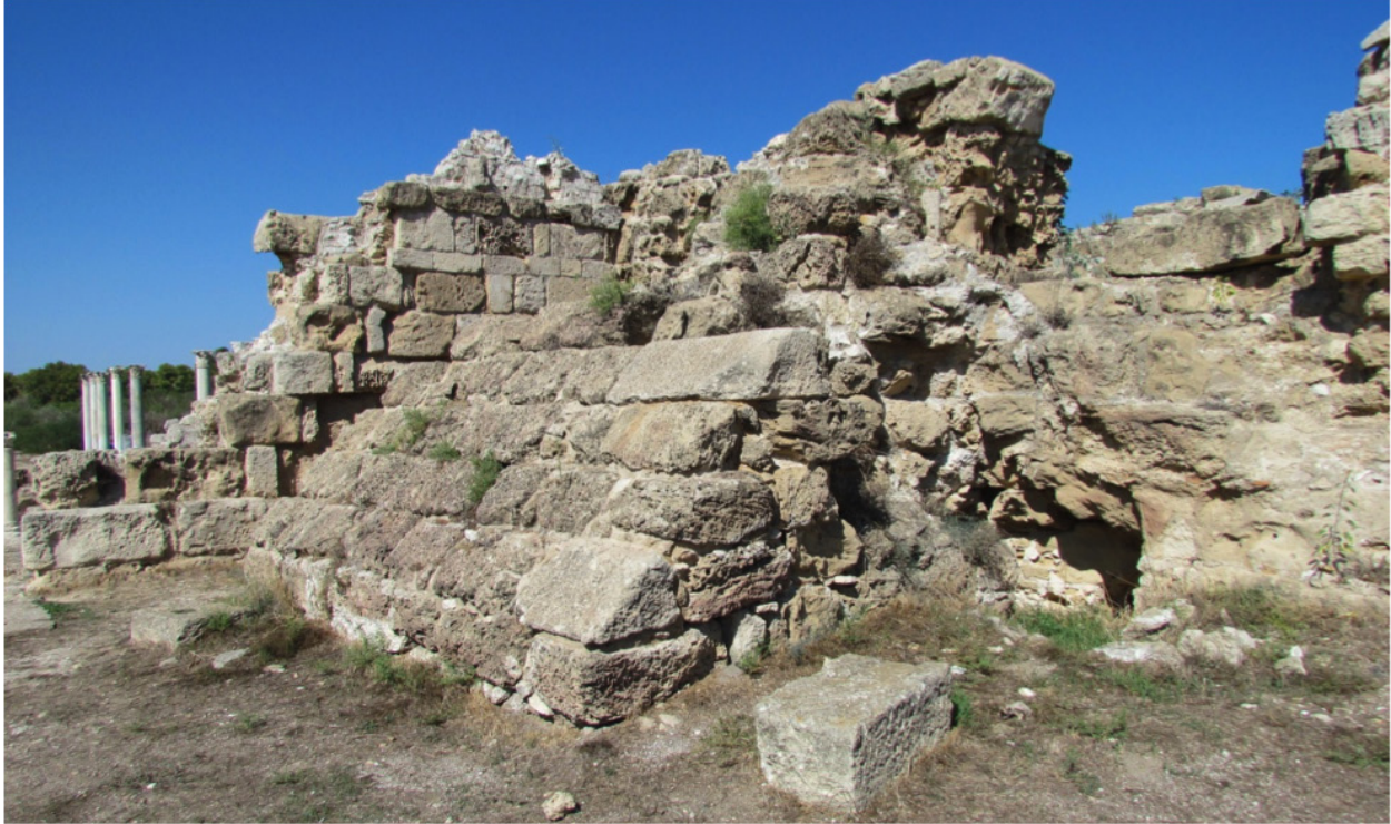
Fig. 8: Grand Baths at Salamis-Constantia. Massive pier-buttress on the exterior of the south frigidarium.
