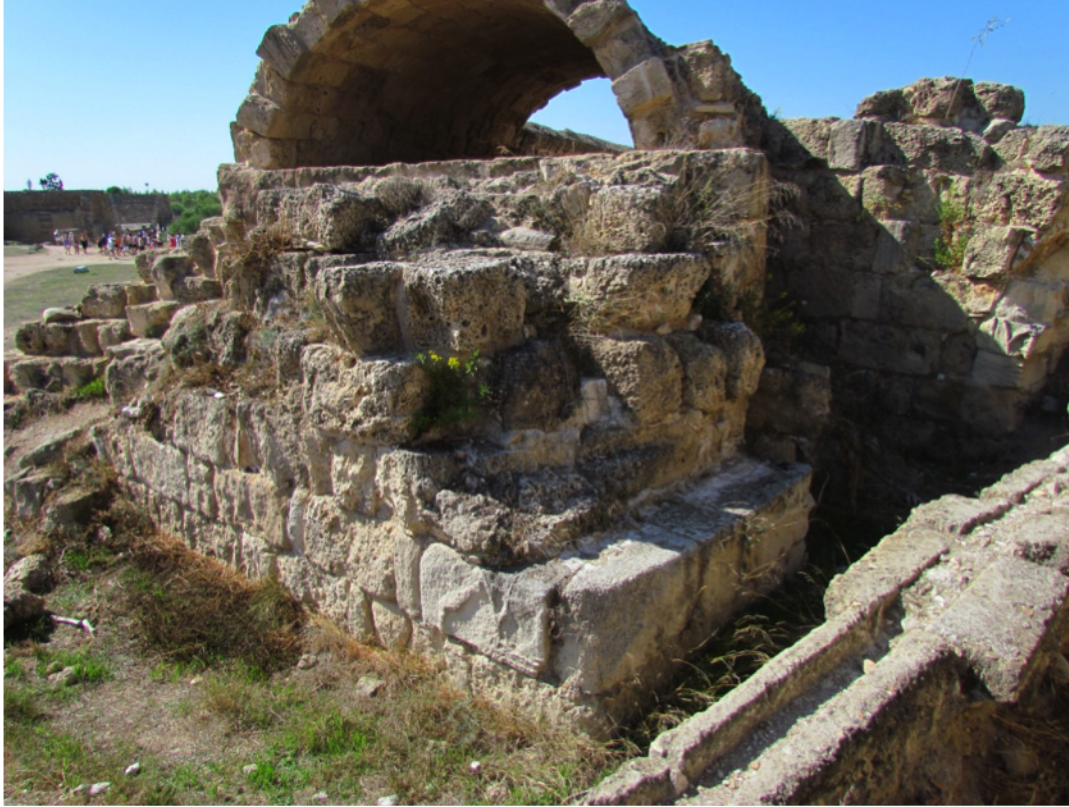
Fig. 9: Grand Baths at Salamis-Constantia. Remains of the flying buttress on the exterior of the south sudatorium, east of the cistern. Notice the water channel underneath.
