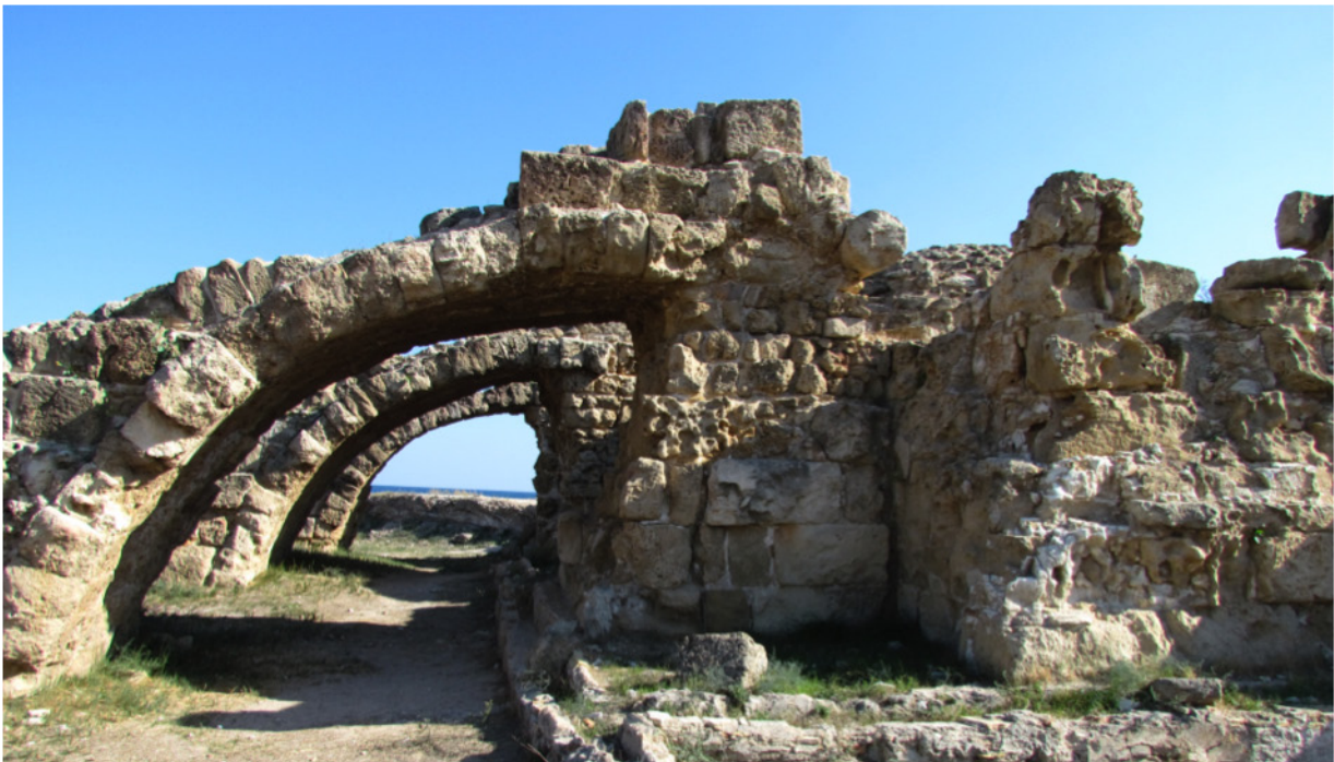
Fig. 7: Grand Baths at Salamis-Constantia. Exterior of north wall showing the water channels running beneath the flying buttress.
