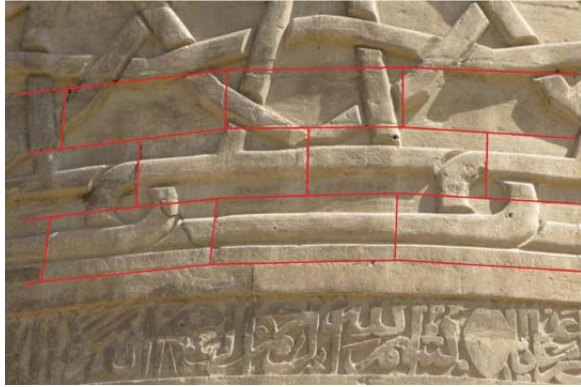
Fig. 11: Detail of Barsbay dome (photo: authors)
