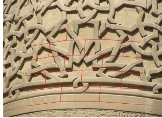
Fig. 12: Detail of Ganibek dome (photo: authors)
