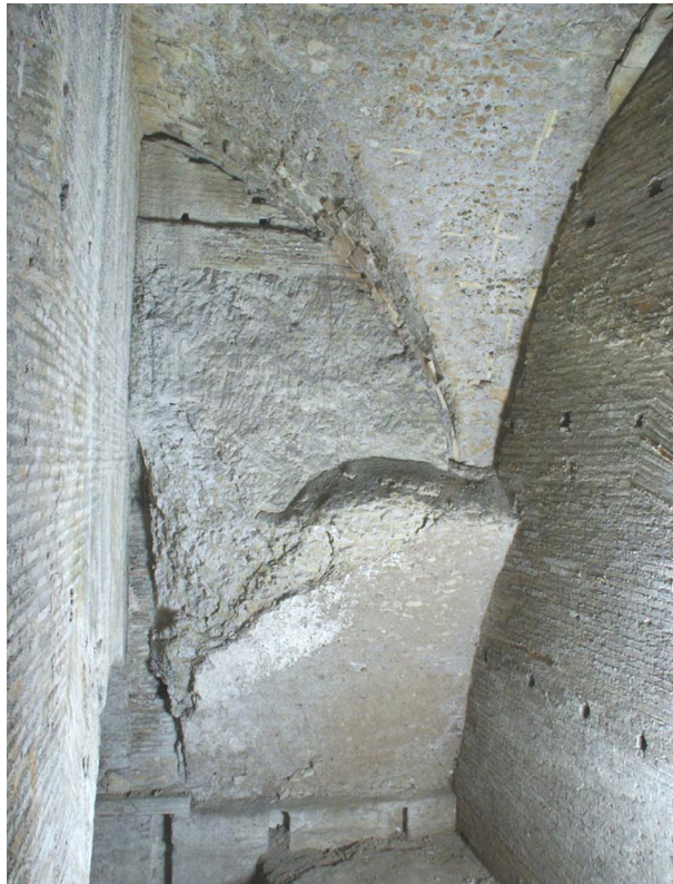
Fig. 11: 'Domus Severiana'. Upper-storey. Coffered flavian barrel vault replaced by a groined vault in severian time.
