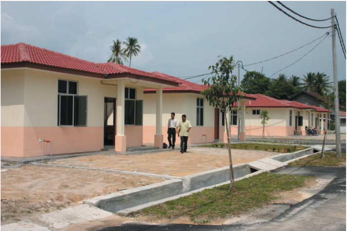
Plate 4 New housing adjacent to Sungei Ranggor Besar in Kuala Teriang, constructed to replace housing destroyed by the tsunami
