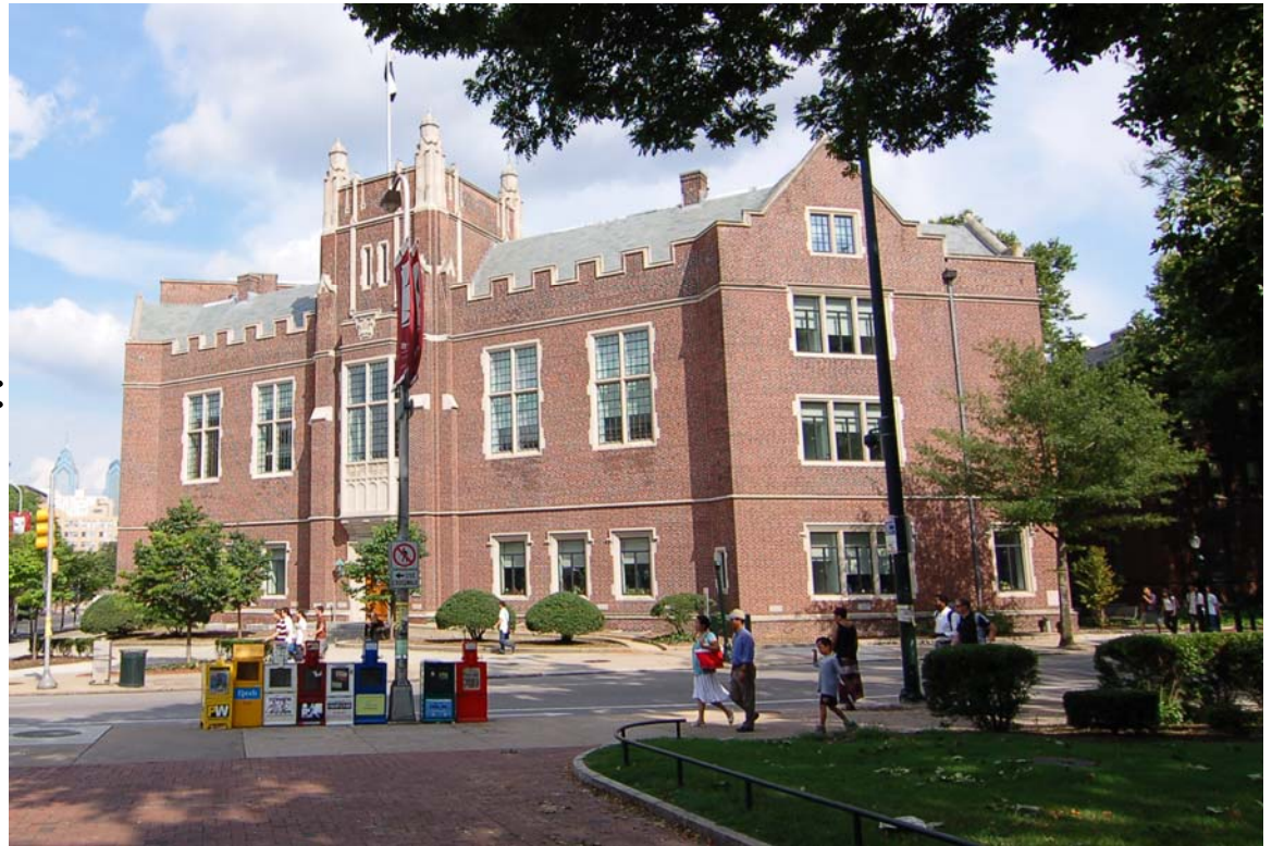
Photo- Fisher-Bennett Hall, location of the ELP at 34th and Walnut Streets
