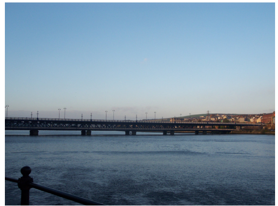
Craigavon Bridge - Derry/Londonderry
